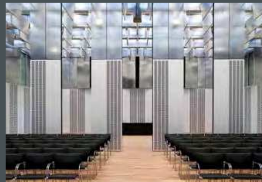
Sheet Steel The metal is impact and scratch resistant. It is always in B1 quality (difficult to ignite) and also magnetic over the whole surface
